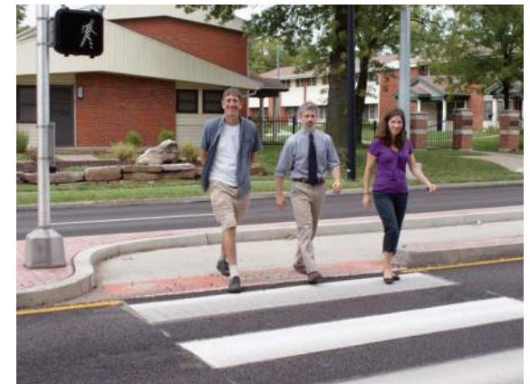
Signalized Mid-block Crossing with Offset Median Refuge Island
